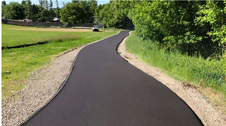
Pathway & Sports Court Rehabilitation
